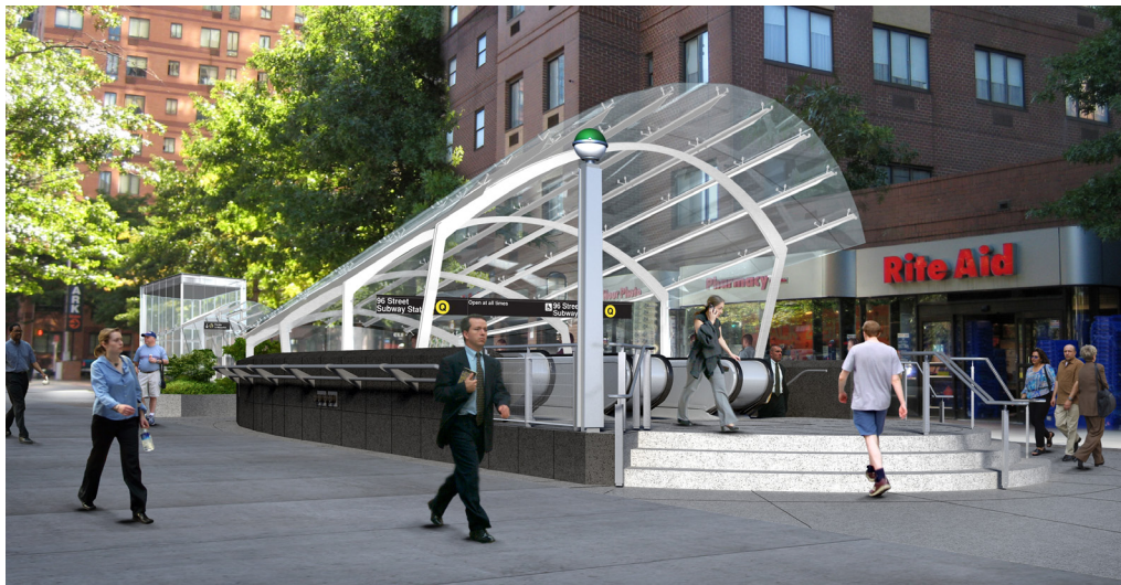
Future entrance of the 96th Street Station on Second Avenue.
