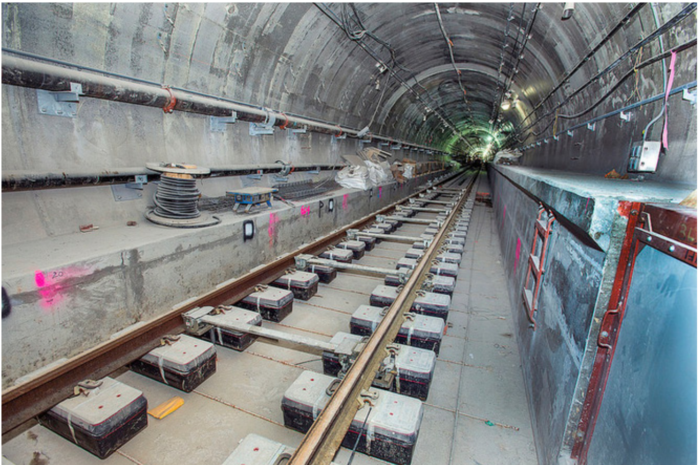
Track in place (91st Street Looking South)
