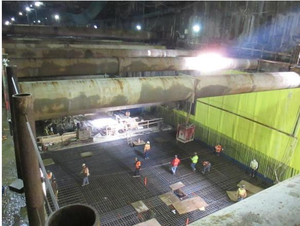
Installation of rebar (reinforcing steel) for the invert slab in the main station
