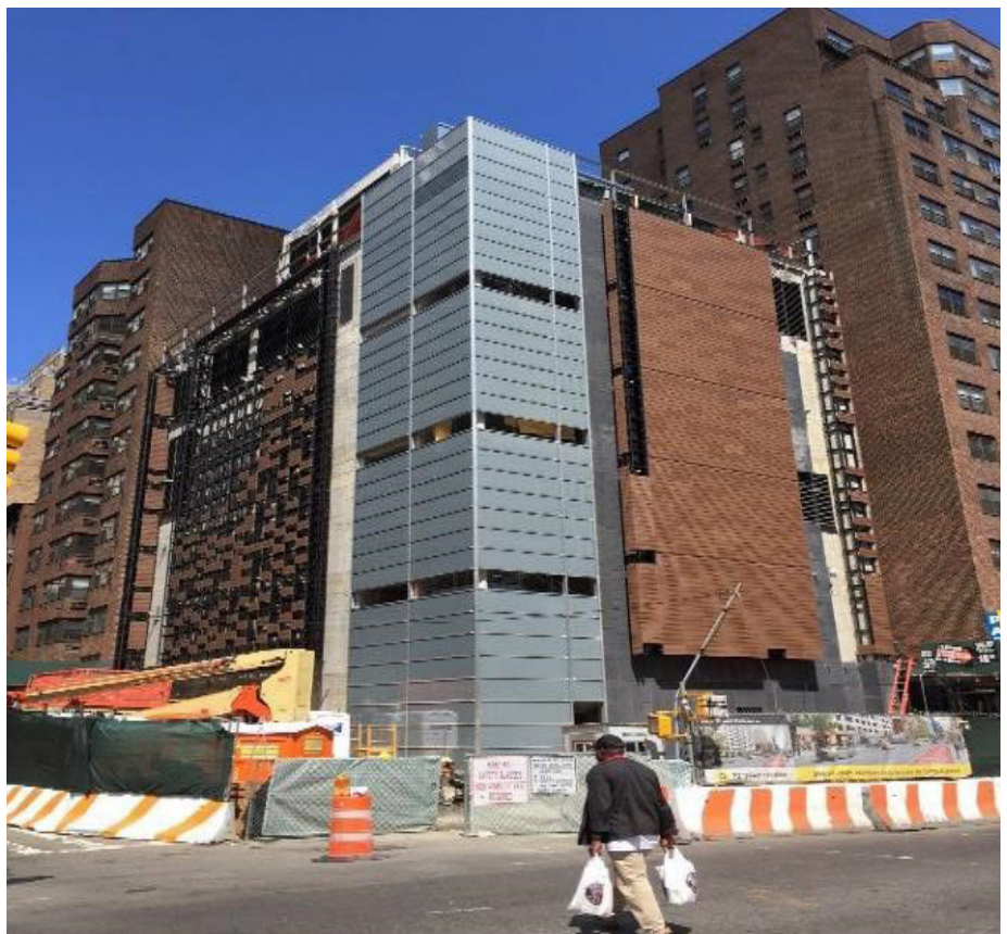
Ancillary 1 (NW corner of 69th Street and Second Avenue) façade installation
