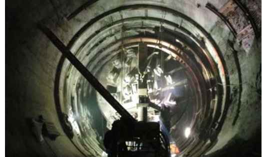
TBM being removed from the West tunnel via a dolly system
